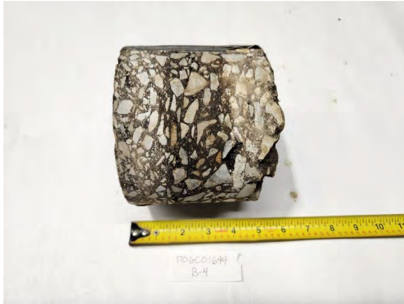
Figure B-4.3 Recovered Pavement Core
