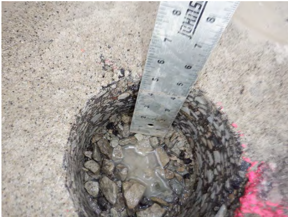
Figure B-5.2 Downhole View
