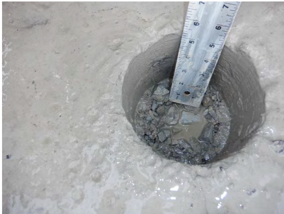
Figure B-9.2 Downhole View
