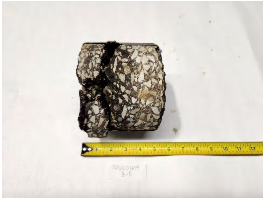
Figure B-5.3 Recovered Pavement Core
