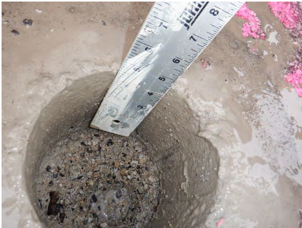
Figure B-7.2 Downhole View
