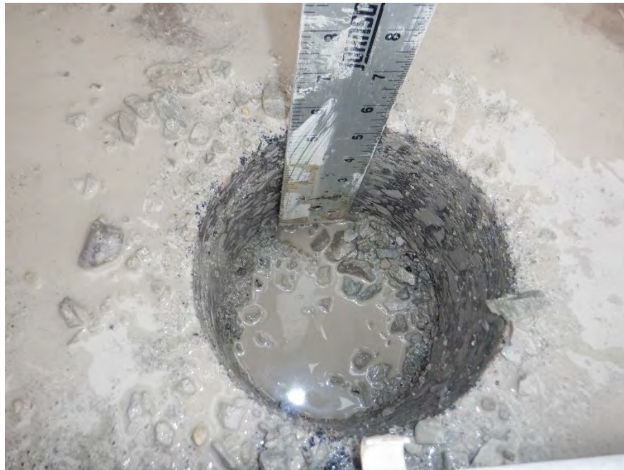
Figure B-13.2 Downhole View
