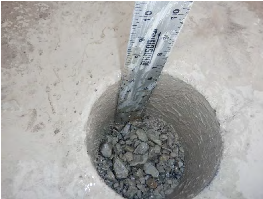
Figure B-10.2 Downhole View
