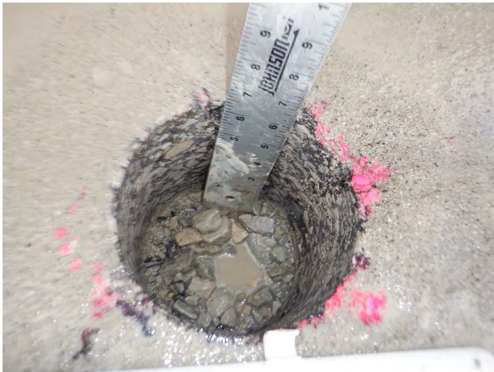
Figure B-2.2 Downhole View
