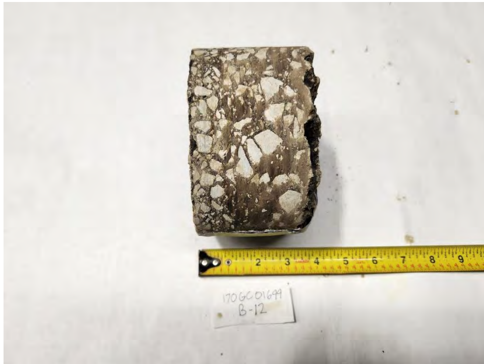
Figure B-12.3 Recovered Pavement Core
