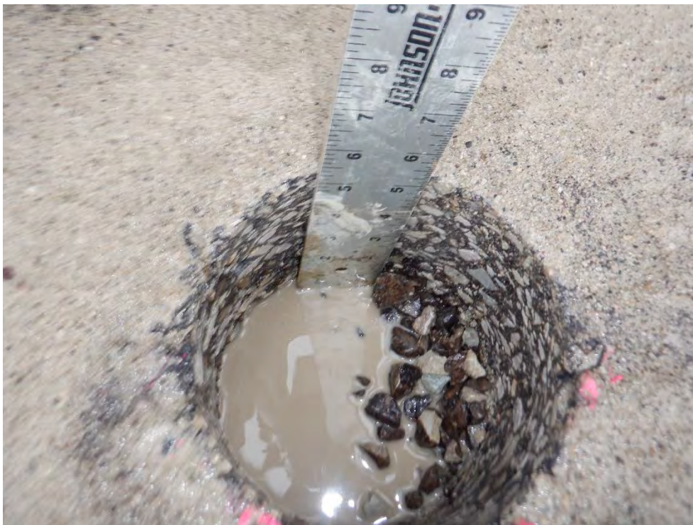
Figure B-1.2 Downhole View
