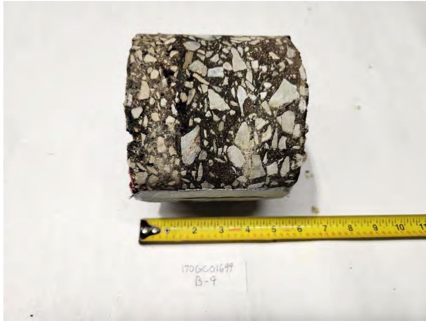
Figure B-9.3 Recovered Pavement Core
