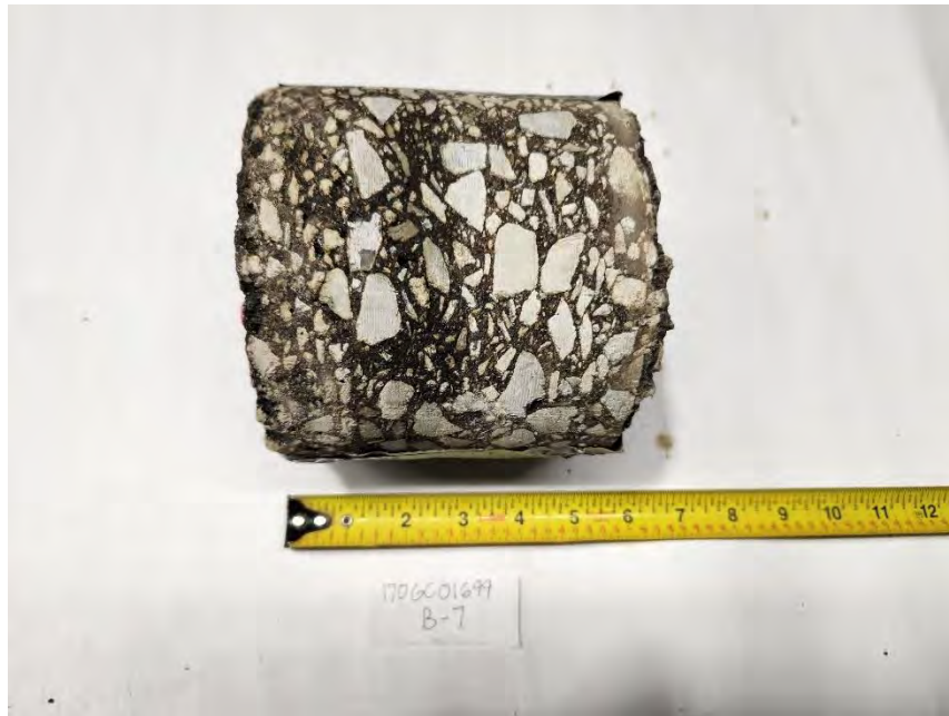
Figure B-7.3 Recovered Pavement Core
