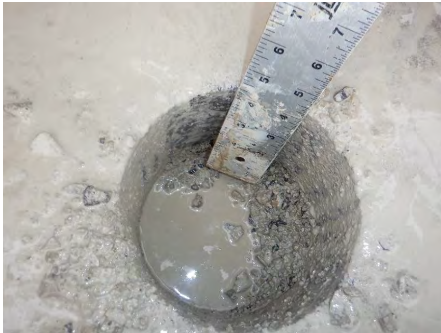
Figure B-11.2 Downhole View
