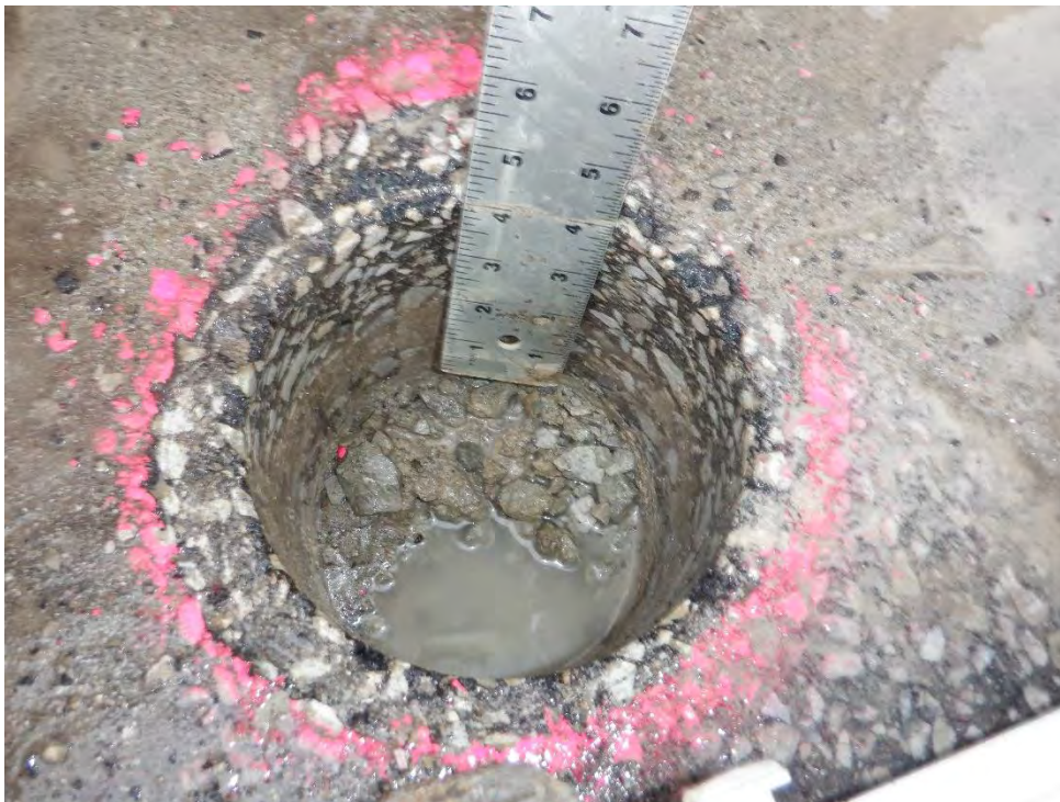
Figure B-6.2 Downhole View
