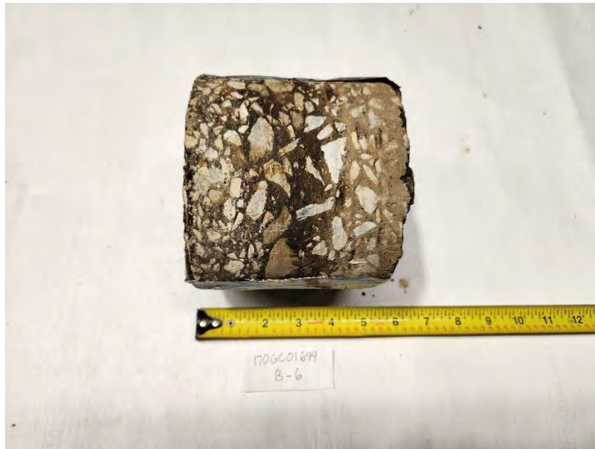
Figure B-6.3 Recovered Pavement Core
