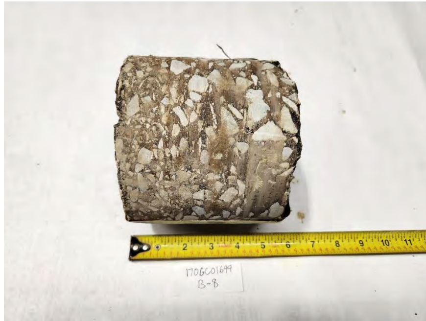
Figure B-8.3 Recovered Pavement Core
