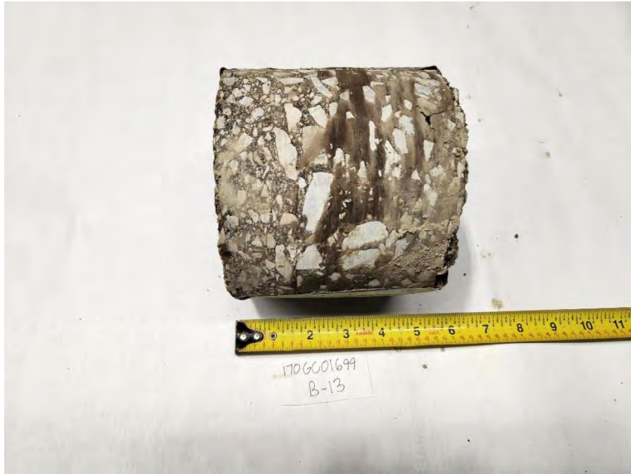
Figure B-13.3 Recovered Pavement Core
