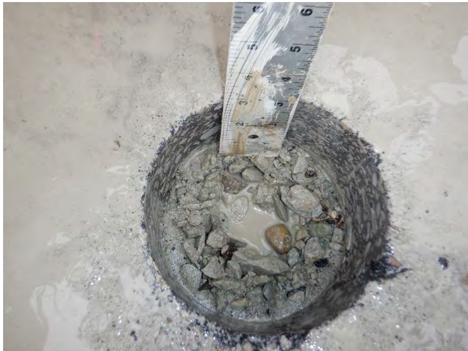
Figure B-12.2 Downhole View
