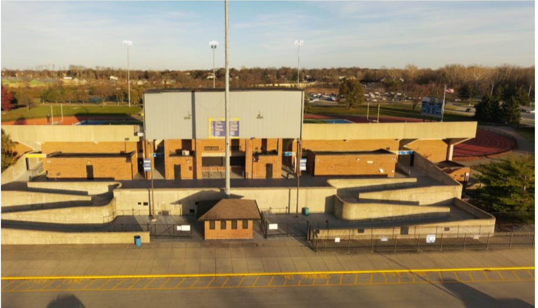
Carmel High School Football Stadium Addition & Renovations
