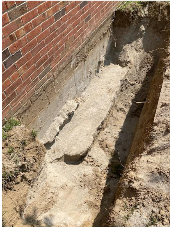
Foundation at Location TP-1
