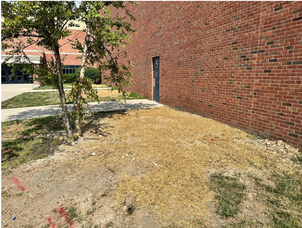
TP-1, 3, and 4 Restoration
