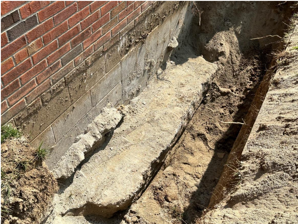
Foundation at TP-1
