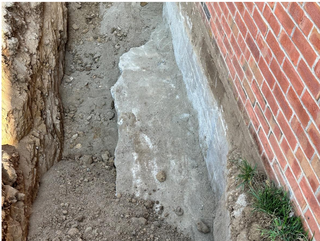
TP-3 Looking West
