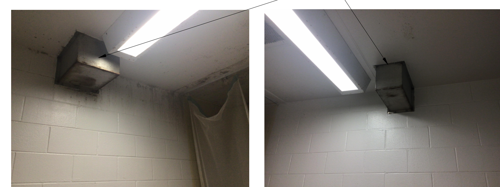
3 STAINLESS STEEL BULKHEAD COVER - TYPICAL SCALE: N.T.S.
